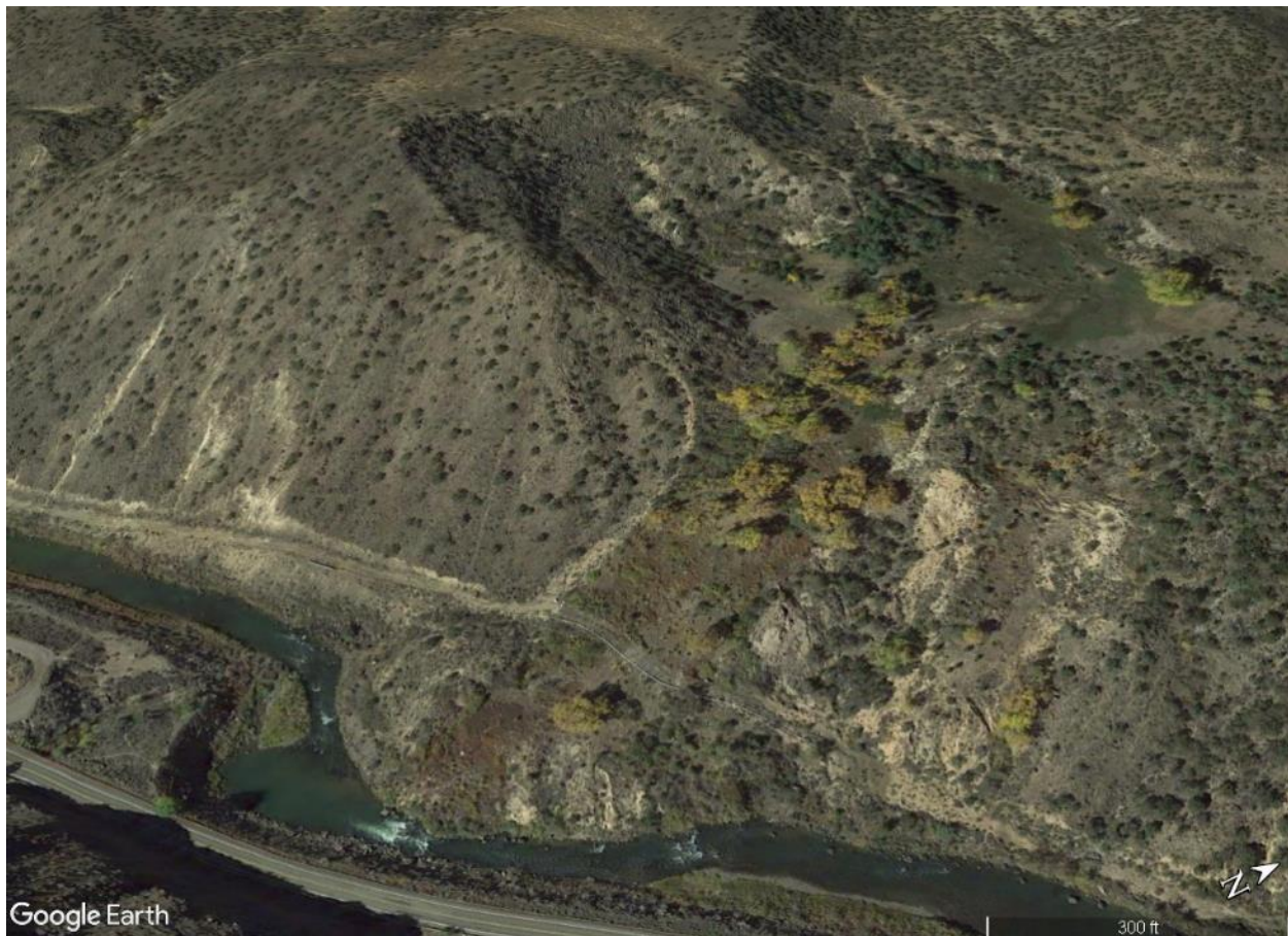
Figure 6-102 Google Earth Image Showing an Active Landslide in New Mexico
