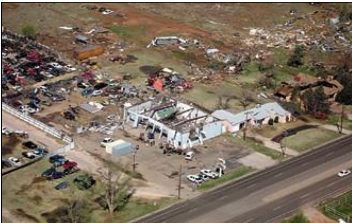
Figure 6-145 Clovis Tornado Damage
