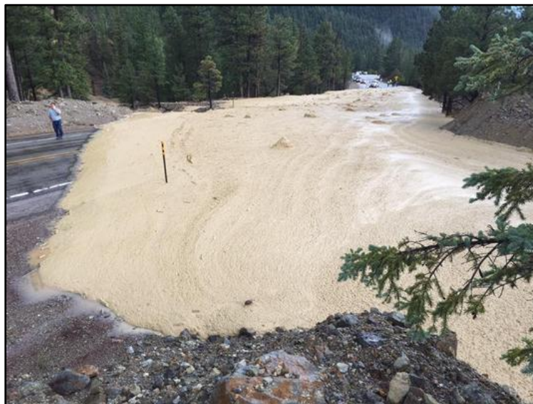
Figure 6-109 Mudslide Occurrence on Highway 38 in Preparedness Area 3
