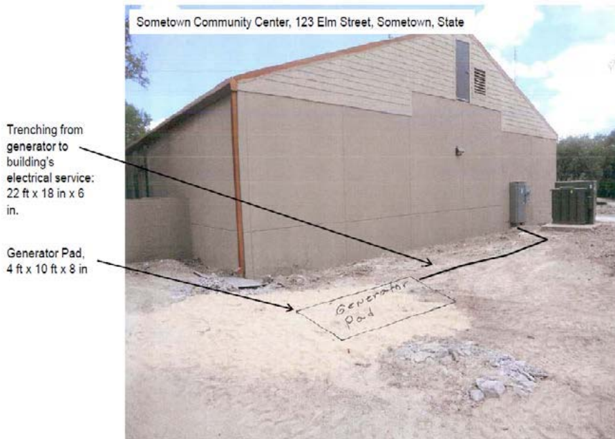
Figure 4. Ground-level photograph showing proposed ground disturbance area.
